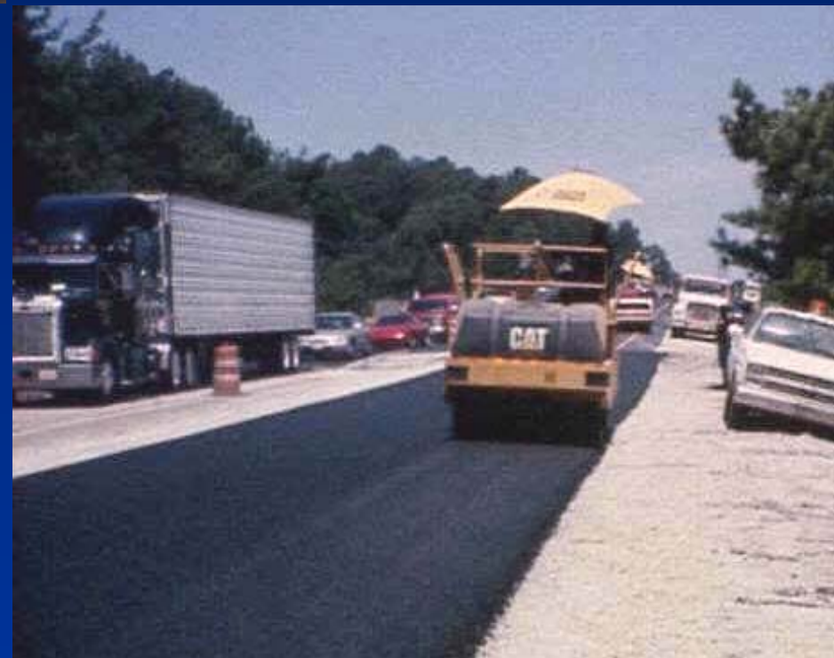
I-40 PCC Stabilization, Overlay N. Little Rock, AR
